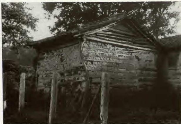
FIGURE 6.— Twisted guachipilin horcones support a bahareque dwelling (photo by Scott Brady).
